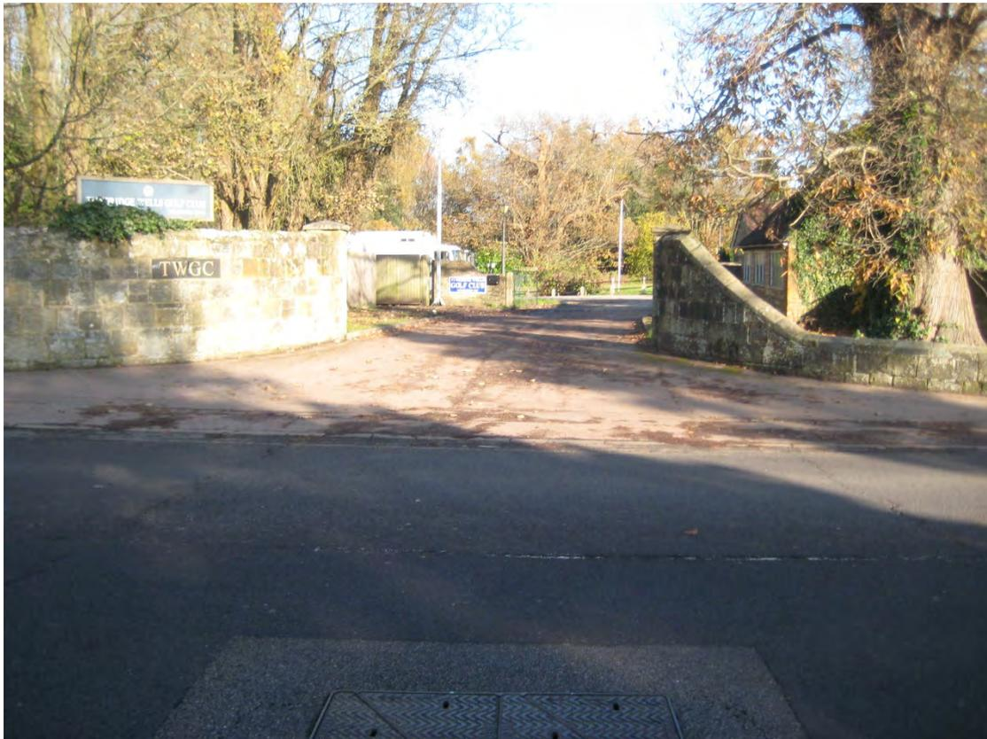
The A264 adjacent to the Site is a primary distributor road operating under a street lit 30mph speed limit. It has an 8.5m carriageway width and a footway to the north on the site side ranging between 2-3.2m in width. Double yellow line restrictions are present on both sides. Further east and west from the Site are pedestrian crossing refuge islands and central hatching areas providing crossing points to footways that are introduced on the southern side further away from the site.
